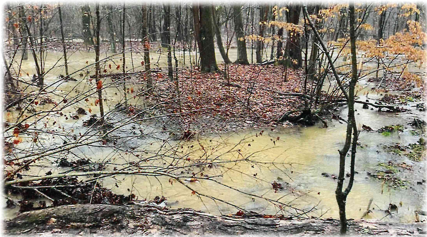
Large wood installation allows high water to be spread across Higgins Run floodplain.
