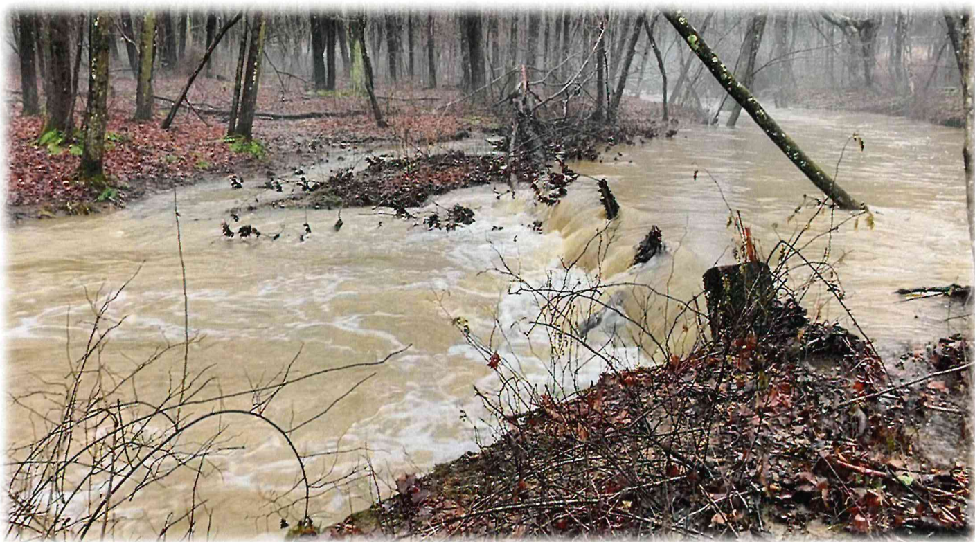
Large wood structure reduces stream velocity, retains sediment, debris and leaves.
