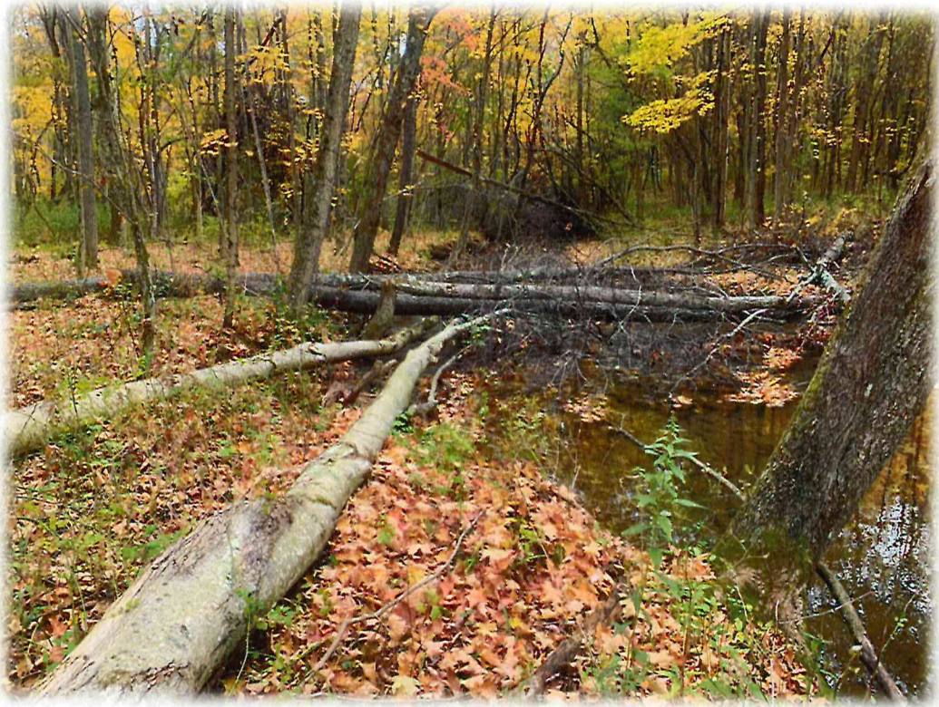
Large wood structure spans stream channel and is “pinned” on each bank to combat movement during high water events.
