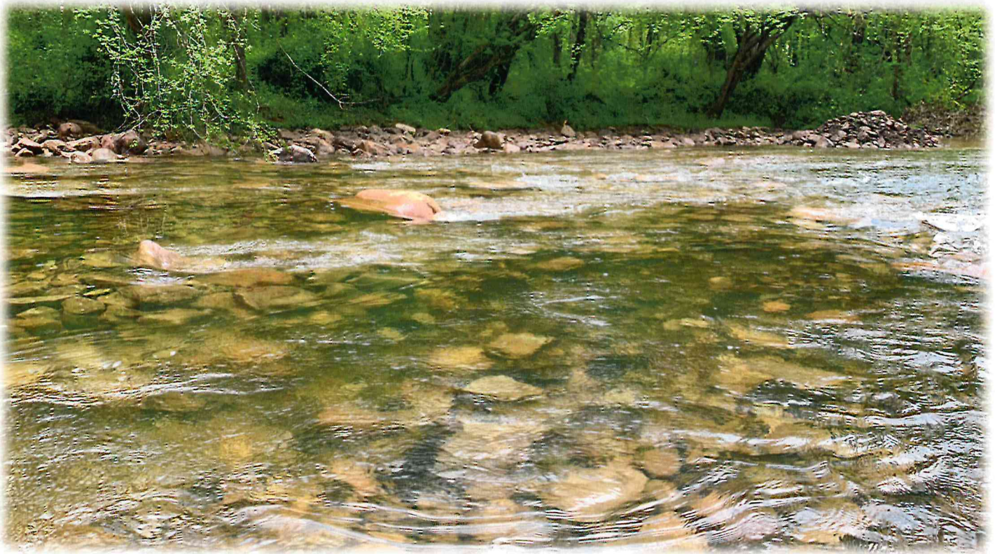
River rock was placed across stream bed to create diverse riffle habitat for fish and other aquatic life.
