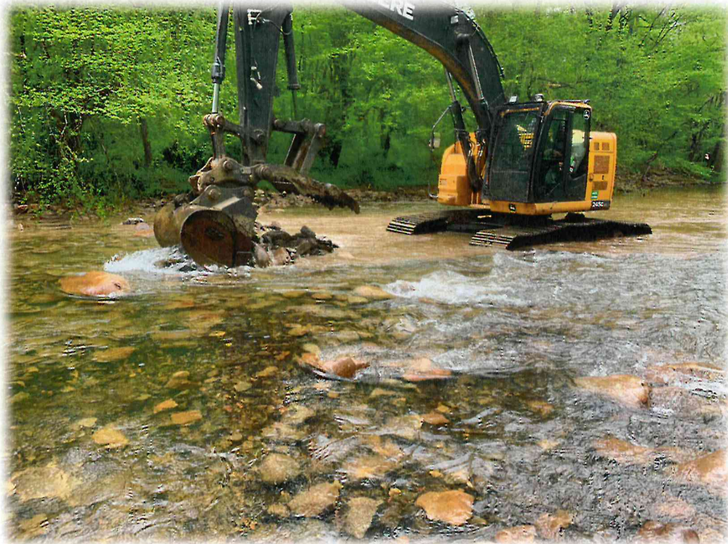
Screened river rock being placed in Quemahoning Creek to create riffle habitat.
